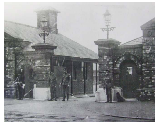
Cavalry Barracks original main entrance c1910
