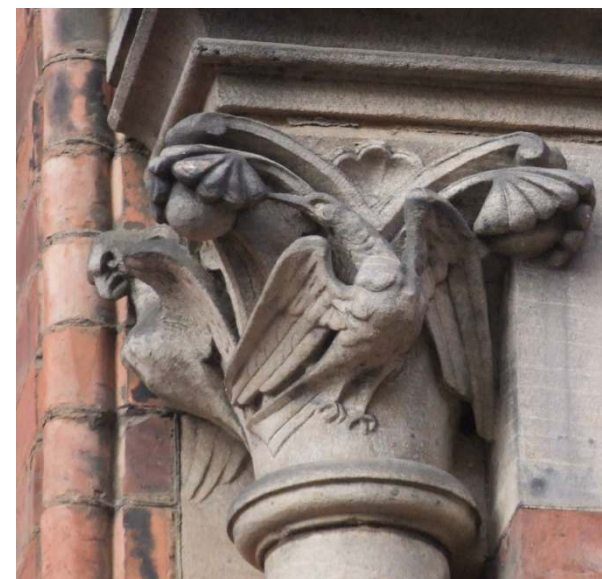
Wenlock Terrace – typical column head
